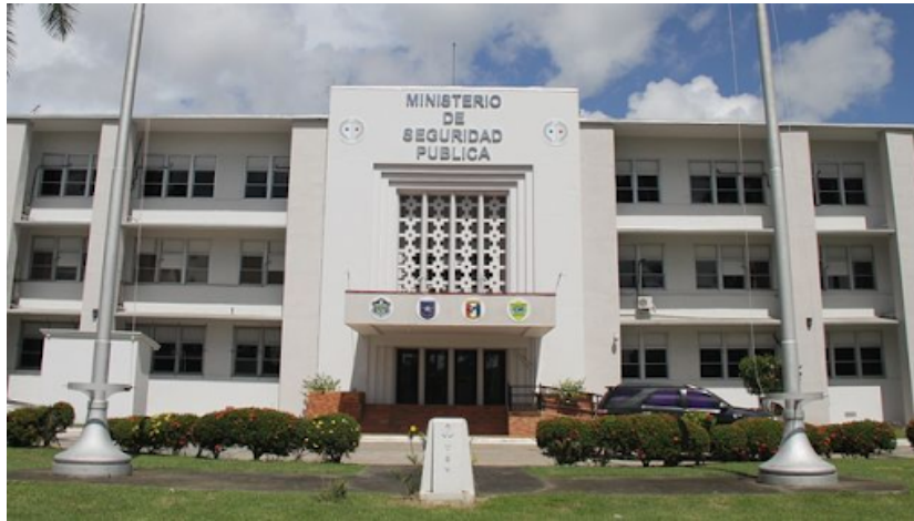
Figure 2: Telemetro. Picture. In the image, the main building of the headquarters of the Ministry of Public Security, in Ancon, Panama City, Panama.
